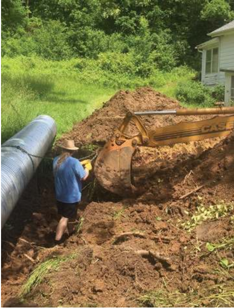
Dennis guiding a new culvert into place.
