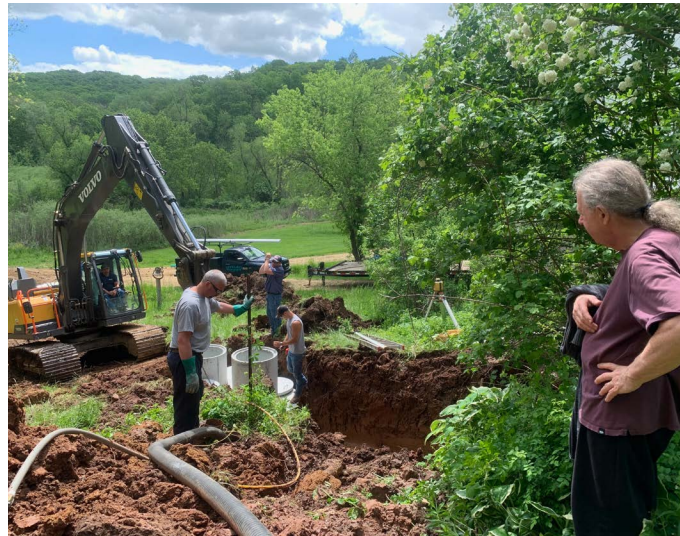
A new septic tank was installed for the farm house.
